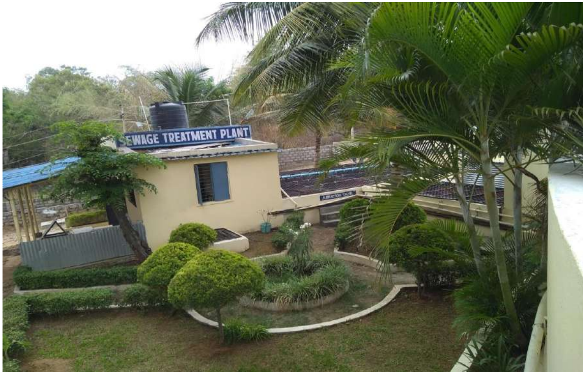
Figure: Waste Water Treatment Systems-250KLD
